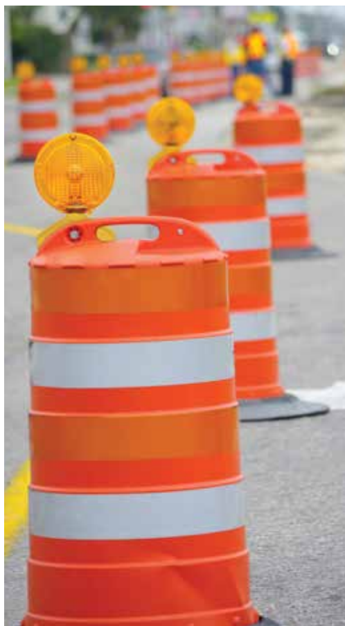
Barricade lights at construction site.
